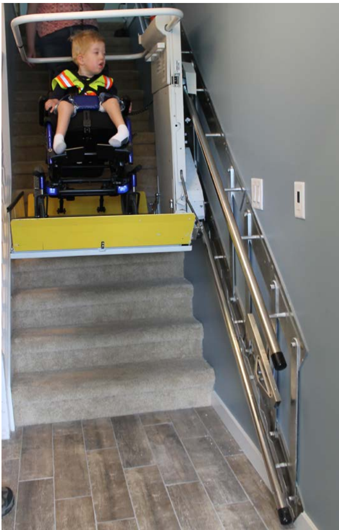
Jack Cholette takes a ride on his newly installed stair lift.
